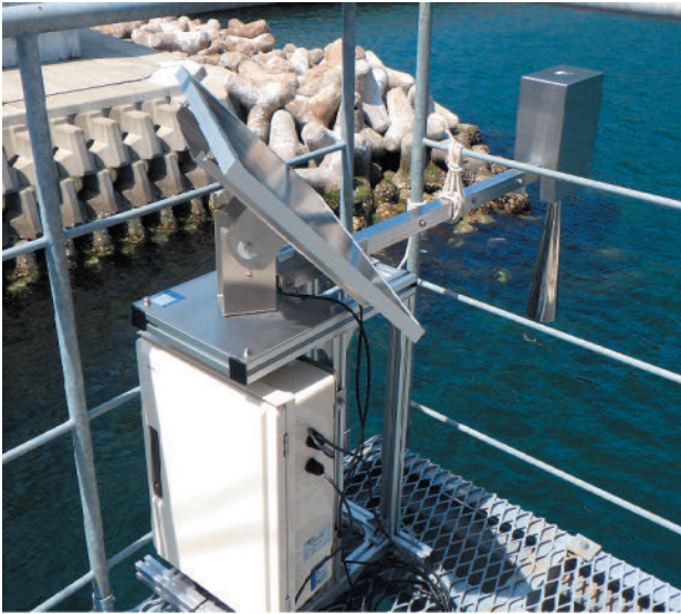
Photo 4. Portable radio wave-type installed outside the Kamaishi tide station.
